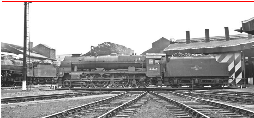
Royal Scot Class 4-6-0 No.46169 The Boy Scout is pictured on August 18th, 1962 on the turntable outside the semi-roundhouse at Crewe North Shed . The construction of the roof for the semi-roundhouse – which was completed in 1959 – must have been one of the last significant enhancements to a steam locomotive shed.
