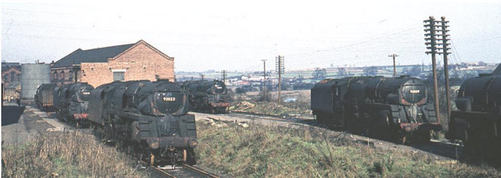
This photograph of **Wellingborough Shed Yard** on February 7th, 1960 shows six of the seven Crosti-boilered 9Fs in store prior to their conversion at Crewe Works to a conventional boiler. Three can be identified as 92021, 92022 and 92029. *Colour-Rail 100698*
